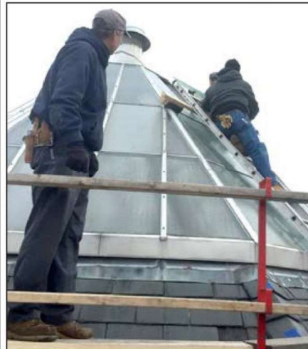
Workers are shown repairing the atrium recently.
